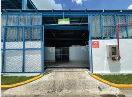
WWTP of Vietnam facility
