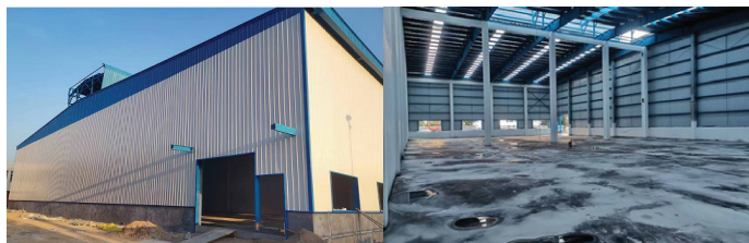
Brand new Class C chemical warehouse
