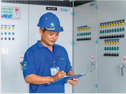
WWTP of Vietnam facility
