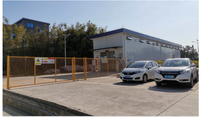
In our China facility, we installed a fence to prevent unauthorized outsiders from entering the Hazardous Chemical Warehouse
